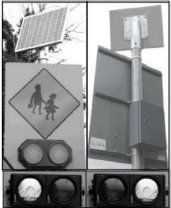
The electrical energy is then changed into a form of energy that can be stored in a battery.
